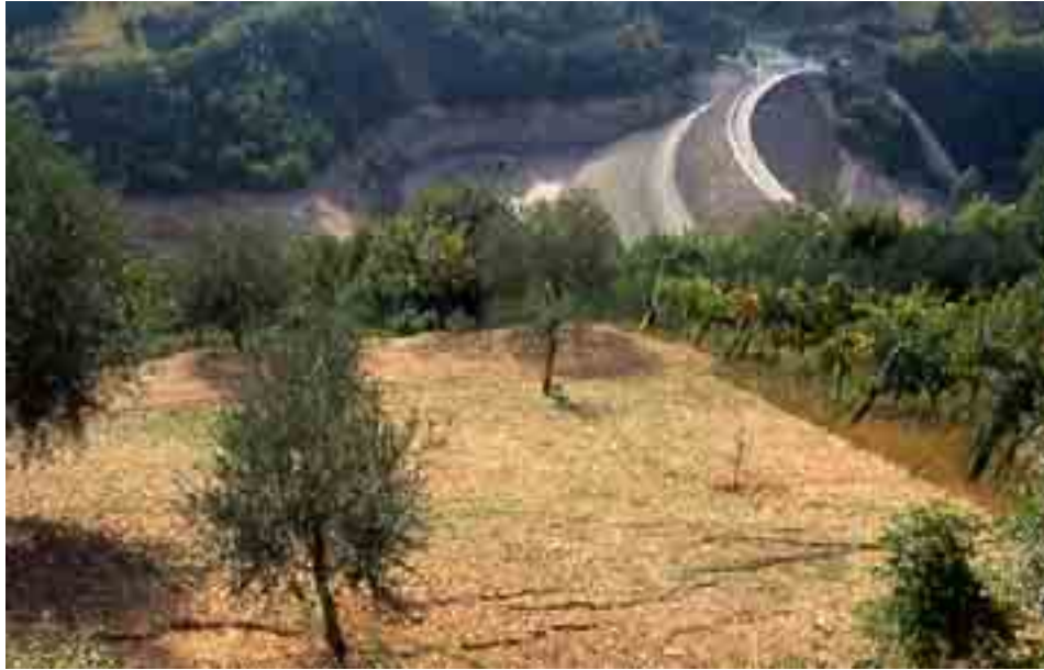
Figure A3.32 – Crown of landslide menacing the emptied Acciano reservoir, induced by the 26 September 1997 Umbria-Marche earthquake ( M_w 6.0). Photo E. Vittori.
