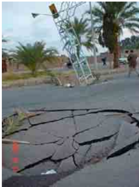
Figure A3.35 – Sinkholes near Bam (southern Iran) following the 26 December 2003 (Mw 6.5) Bam earthquake. The local macroseismic intensity was IX MM (source: Eshghi and Zarè, 2004).
