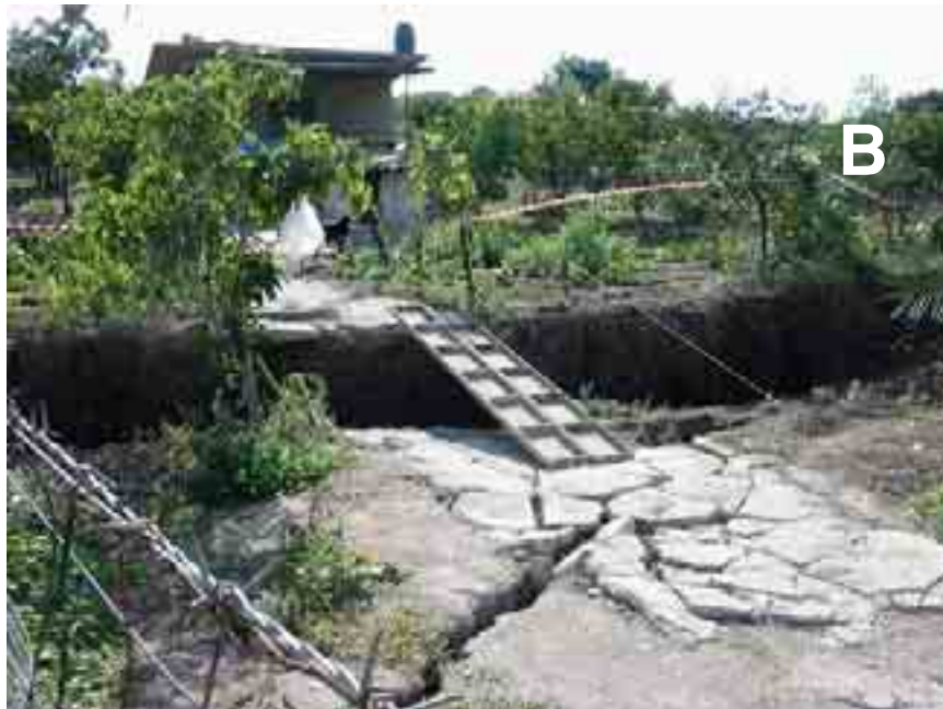
Figure A3.33 – A: flank of a wide landslide occurred near Cerda (Palermo, western Sicily) following the September 6, 2002 (MI 5.6) Palermo earthquake. B: particular of the crown. A local macroseismic intensity of V (EMS98) was estimated at Cerda. Photos M. Guerra and E. Vittori.
