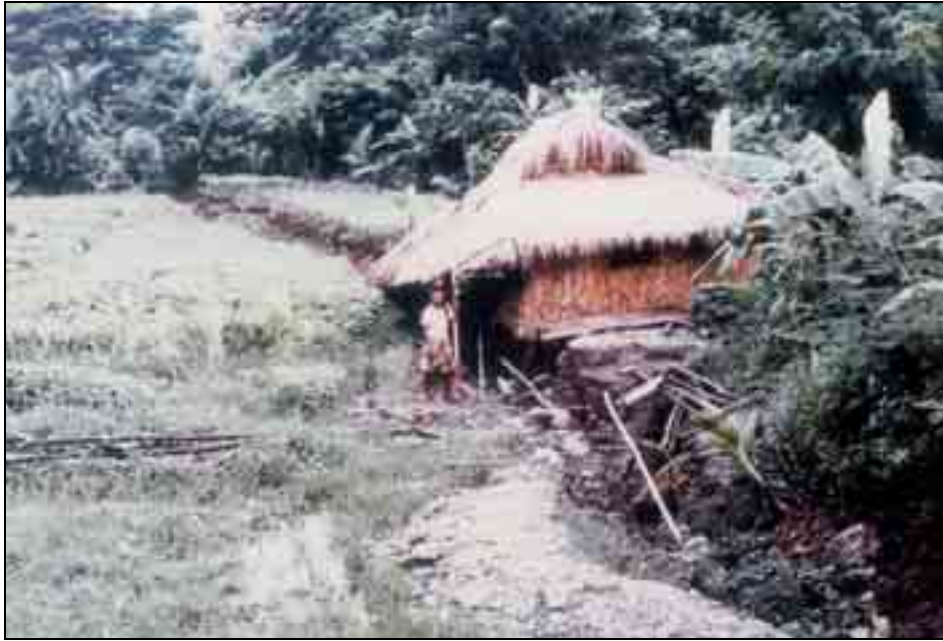
Figure A3.7 – Left-lateral (5m) and vertical (0.7 m) faulting associated to the 16 July 1990 Luzon (Philippines) earthquake ( M_s 7.8) (Yomogida and Nakata, 1994). Photo courtesy of T. Nakata.
