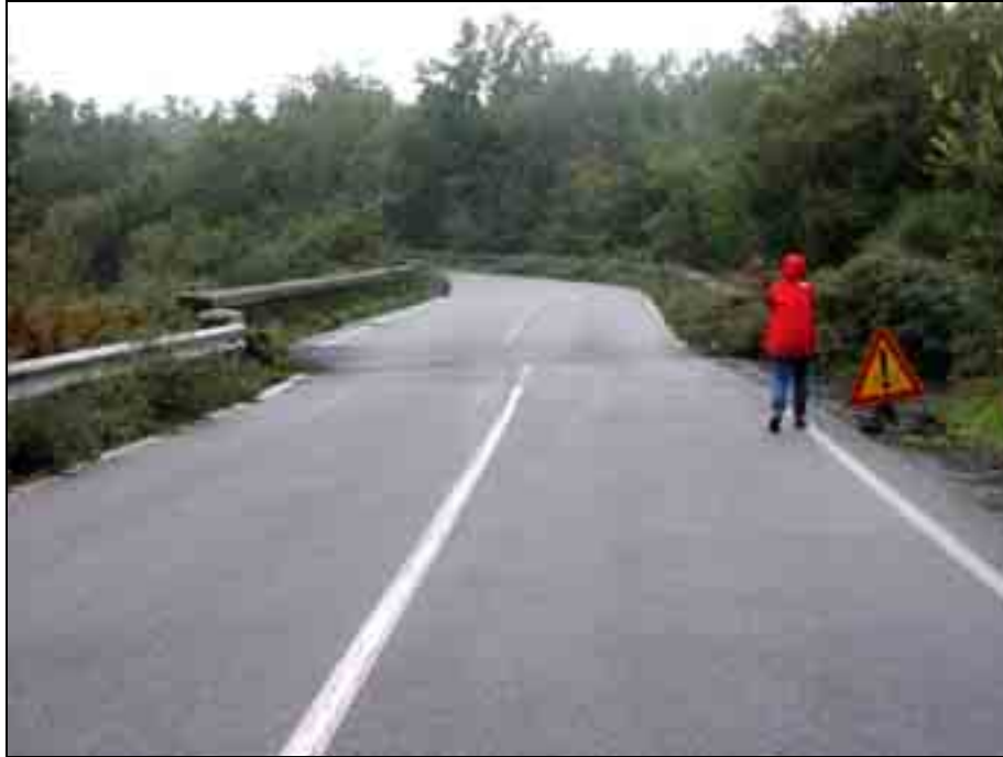
Figure A3.20 – Left-lateral faulting in the eastern slope of Etna volcano (Pernicana fault). Different segments of this fault move either by creep or stick-slip. More than half a meter of slip took place here during the october-november 2002 volcanic and seismic crisis. Photo E. Vittori
