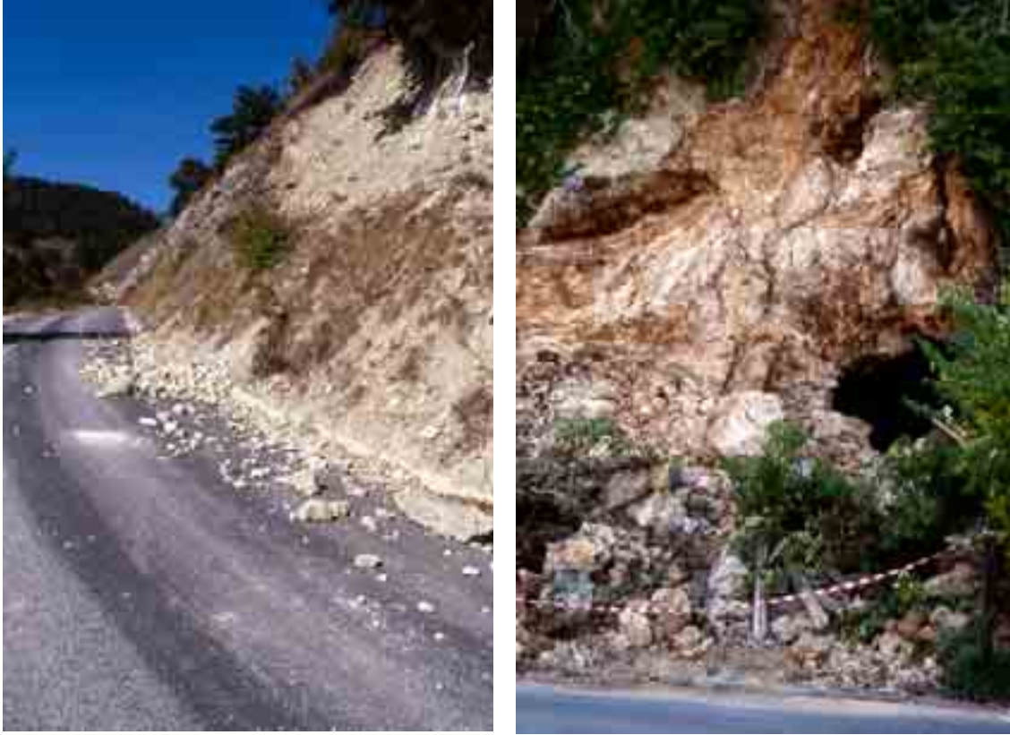
Figure A3.36 – Minor rock falls from the flanks of paved roads near the epicentral area of the 1997 Umbria-Marche earthquake. The preliminary estimate of the Inqua EEE Intensity is VII. Photos E.Vittori.
