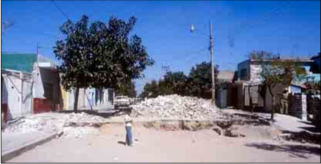
Figure A3.21 – September 19, 1985 Michoacan (Mexico) earthquake (M s 8.0): scarp due to differential compaction in Mexico City. Photo E. Vittori.
