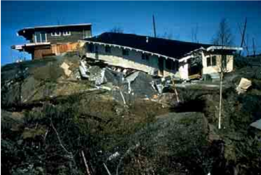
Figure A3.29 – Liquefaction of soil and lateral spreading of saturated soft clay and sand in Anchorage during the Alaskan Earthquake of March 27 1964 (M 8.6). The ground dropped on the average of 11 meters and houses slid about 150 to 180 meters. This effect, which determined a widespread change of the landscape, can be evaluated of Intensity XII in the Inqua EEE Scale. Source: http://cee.uiuc.edu/sstl/education/liquefaction/
