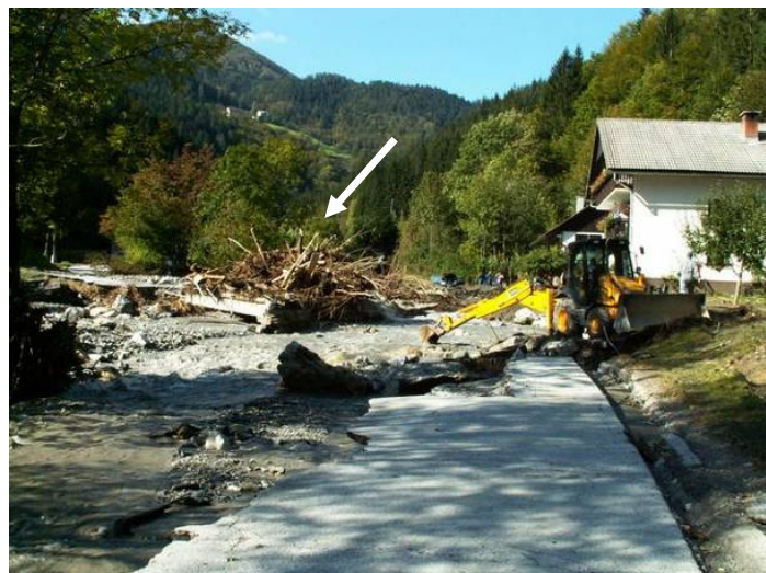
Figure 1. Flash flood in the Davča basin (Slovenia, September 2007). Driftwood and aggradation clogged the bridge (arrow), causing channel avulsion and thus damages to the house on the right of the picture ( http://www.davca.si )
