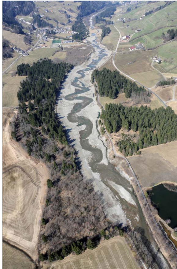
2010 when the works were finished
