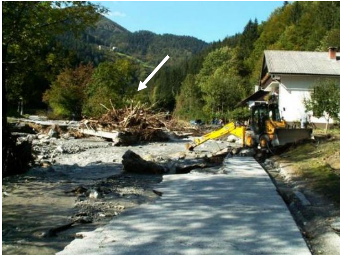
Figure 1: Flash flood in the Davča basin (Slovenia, September 2007). Driftwood and aggradation clogged the bridge (arrow), causing channel avulsion and thus damages to the house on the right of the picture ( http://www.davca.si/ ).
