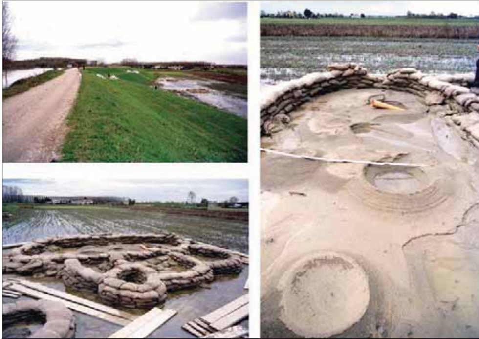
Fig. 5 - Embankment underseepage phenomena ( sifonamento and fontanazzi ) along the Po River right bank near Luzzara (RE) during the 2000 flood event (the local hydraulic head was about 4.5 m). 1000m up-current, previously formed sinkholes were completely empty and dry.
