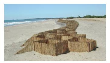
Figure 1.8.2 - Chess-shaped windbreak fences (POSIDUNE, 2007).
