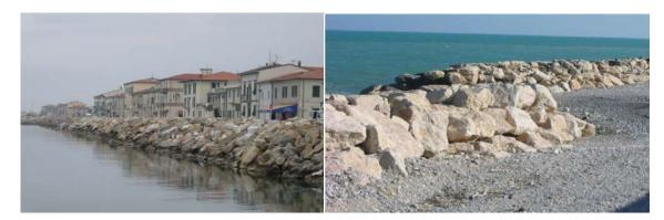
*Figure 1.1.3* – Some examples of riprap breakwaters: to the left, for a urban settlement protection (Photo by ISPRA); to the right, for a shoreline protection (APAT, 2007).
