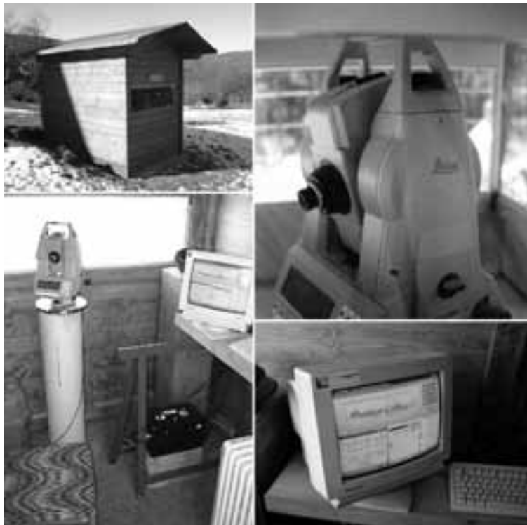
Figure 21 - Poviglio landslide: the automatic motorised theodolite surveys the landslide's movements, enabling villagers to remain in their houses during the construction of the new village in a safer area. Photos by Giovanni Bertolini, September 2003.
