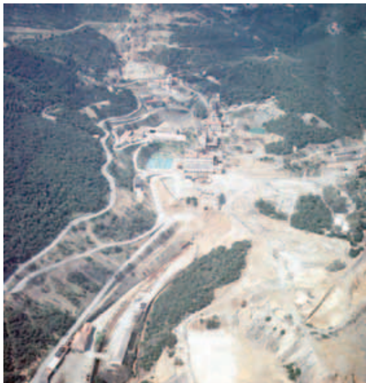
Figure 20 - Aerial view of the Sant'Antonio sector of Montevecchio, showing: excavation at the outcrops of the Sant'Antonio lode (upper part); the Sant'Antonio and Sartori shafts, and the Laveria Principe ore-dressing plant (central-upper part); treatment tailings (lower half).
