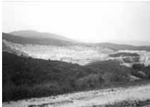
Figure 24 - General view of the Sa Matta talc mine
