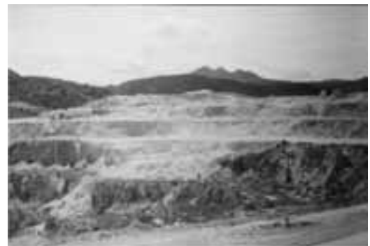
Figure 23 - General view of the Ispaduleddas albitite works
