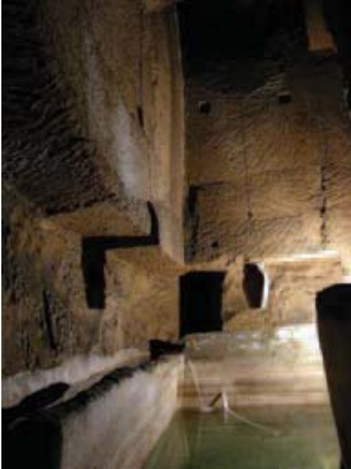
Figure 5.5 - Greek-Roman cisternae: water reservoirs entirely dug in the Neapolitan Yellow Tuff (photo Esposito).
