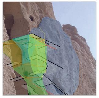
Fig. 8 – Pattern of existing discontinuities at four different stories and reconstructed unstable blocks in the upper East side of Eastern Giant Buddha niche.
