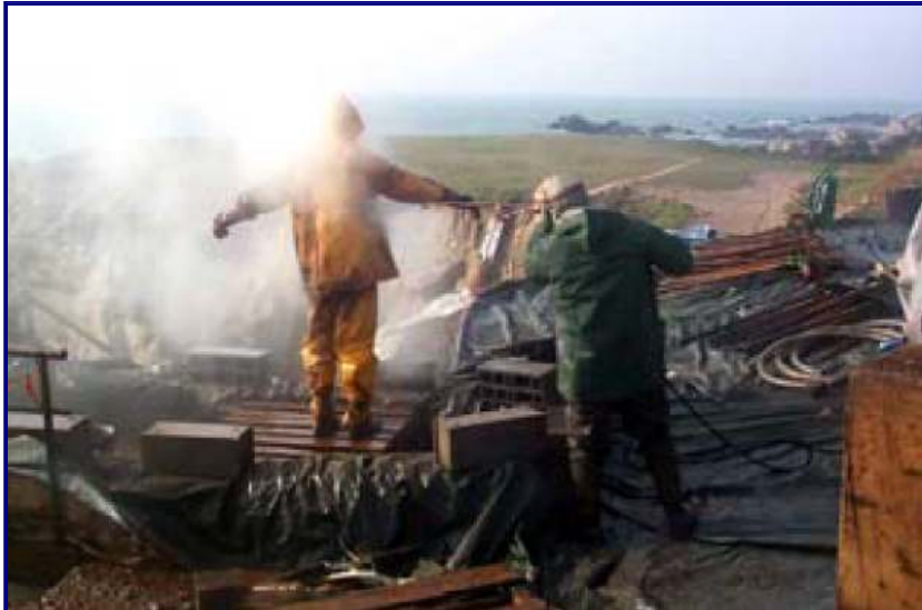
Figure 8. Clean up of personnel once operations are concluded
