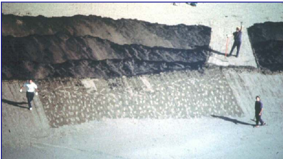
Figure 4. A sandy beach partially cleaned by wooden scrapers (source www.itopf.org )
