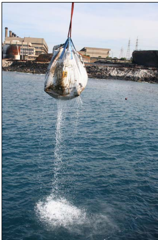
Figure 19: drainage of excess water
