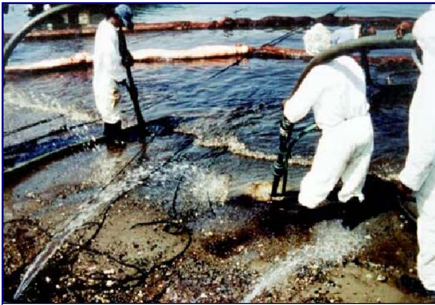
Figure 6. Low pressure flushing of a sandy beach contaminated by buried oil (source www.cedre.fr )
