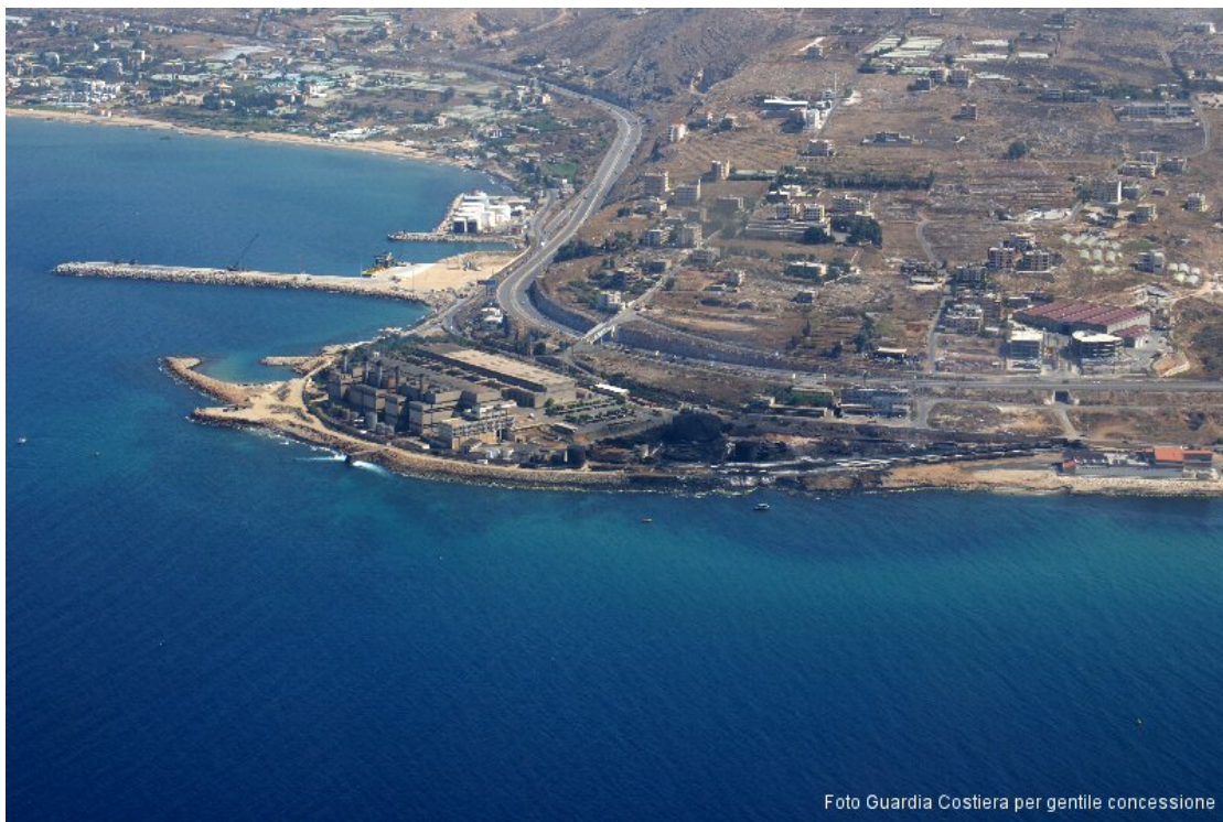
Figure 1 JIYEH Power plant–LIBANON
