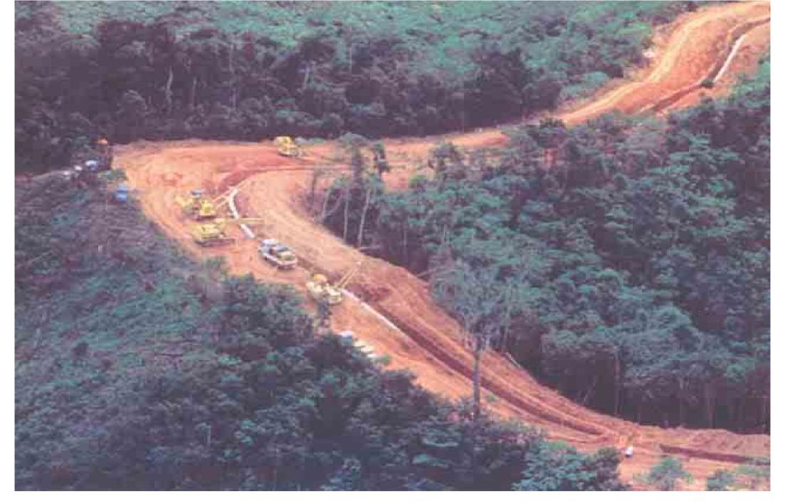
Excavation of the ditch profile to accommodate the welded strings of pipeline
