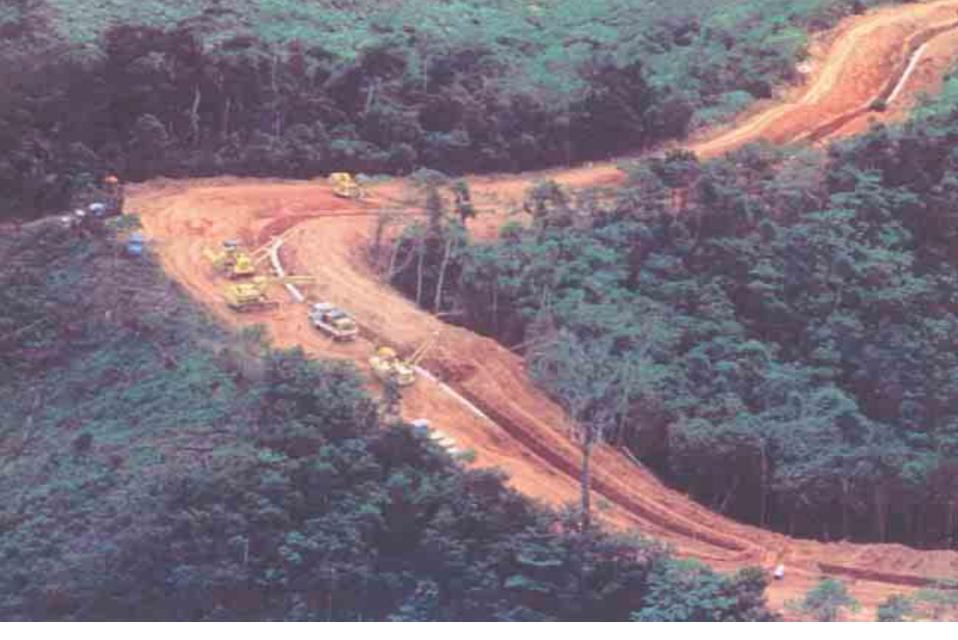
Excavation of the ditch profile to accommodate the welded strings of pipeline
