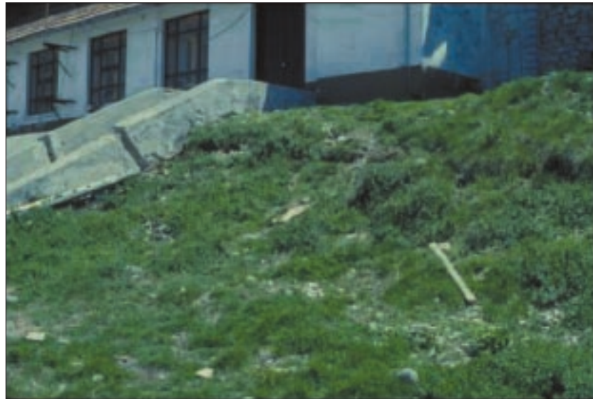
Fig. 8. A ground fracture cutting the stairs of the meteo station at Trevico
