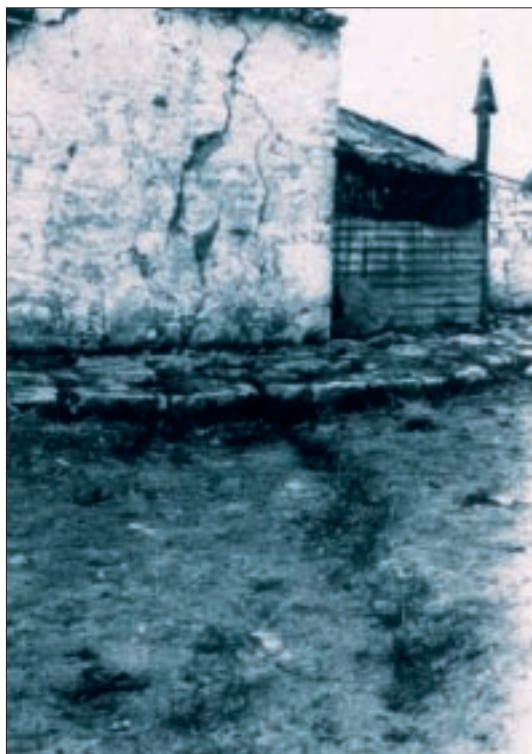
Fig. 2. Earthquake induced ground fracture cutting a house
