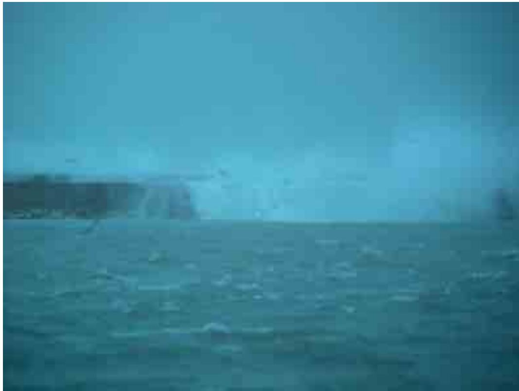
Figure 6: Overtopping of Pescara breakwater by a 4.5 m amplitude wave.
