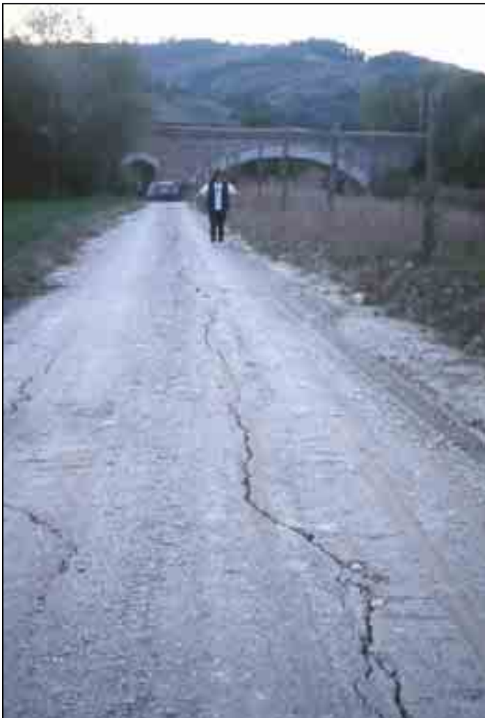
Figure A3.22 – Ground cracks affecting a dirt road in a flat area near Isola (Umbria region), caused by the 1997 Umbria-Marche (Central Apennines) earthquake ( M_w 6.0) (Esposito et alii, 2000; Vittori et alii, 2000). Photo S. Porfido.
