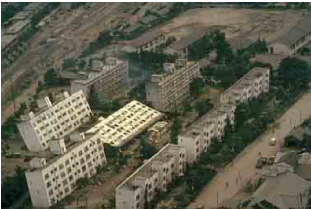
Figure A3.28 – Tilt of buildings at Kawagishi-Cho due to liquefaction following the June 16, 1964 Niigata (Japan) earthquake ( M_s 7.5). The preliminary estimate of the Inqua EEE Intensity is XI. Source: http://cee.uiuc.edu/sstl/education/liquefaction/
