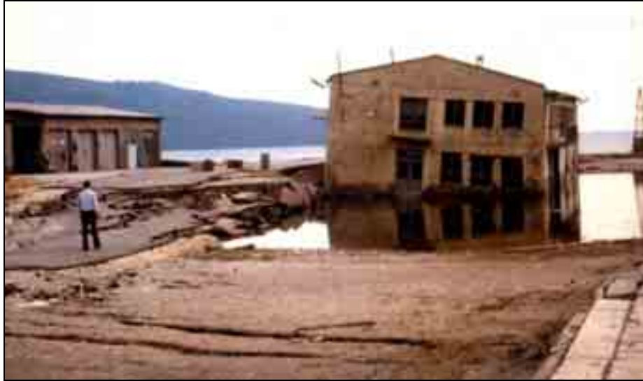
Figure A3.27 – Ground failure (liquefaction of artificial embankment) along the seacoast during the 15 April 1979 Montenegro earthquake ( M_w 6.9). The preliminary estimate of the Inqua EEE Intensity is X. Photo E. Iaccarino.
