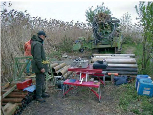
Fig. 21 - a) Continuous boring for CARG 12 survey in Cà Nuova area; b) Continuous boring for CARG 11 survey and gamma ray measurements.
