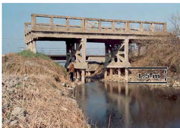
Fig. 94 – A bridge built in 1920s near the southern edge of lagoon at Chioggia, that is now protruding about 1.5 m due to oxidation of surrounding peat soils (from Tosi et alii, 2000).
