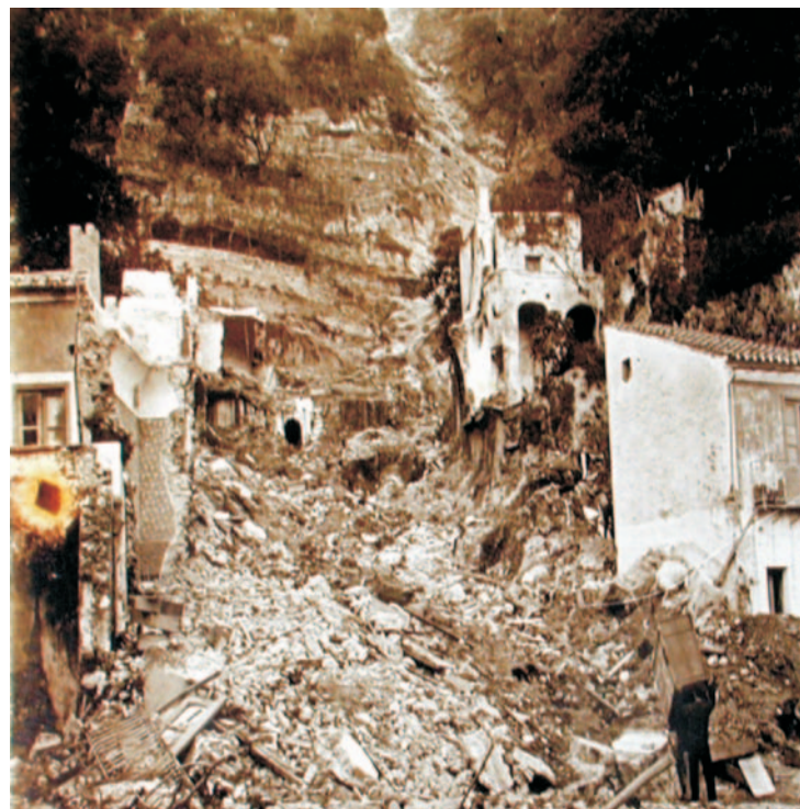
Figure 4: Landslide at Suora Clara, Cetara (Campania Region), 1910
