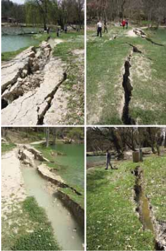
Fig. 6 - Pictures showing the cracks developed after the seismic shocks along the lake shorelines.
