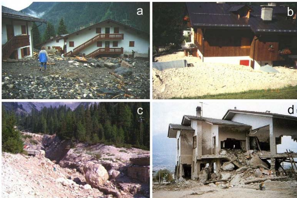
Figure 1. Examples of debris flow damage in Italy: a) Campestrin (Trento, July 1989); b) Cancia (Belluno, June 1996); c) Rudavoi (Belluno, September 1997); Pollein (Aosta, October 2000).
