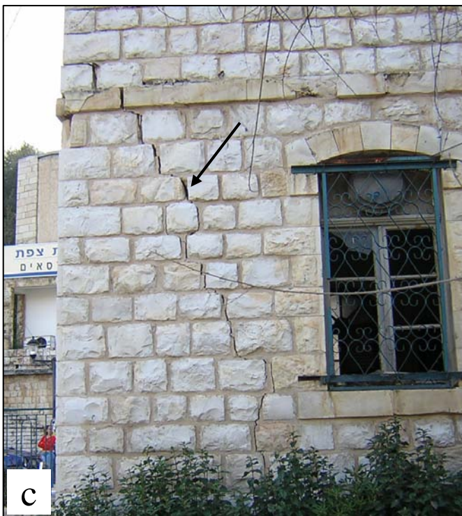
Figure 4: Field evidence for instability of the anthropogenic material slopes. (a) inclined lamp posts found in the anthropogenic talus (marked by arrows); (b) open cracks (marked by arrows) in retaining wall and (c) in building, both found in the anthropogenic talus; (d) rainy winter-season slump in the anthropogenic talus.
