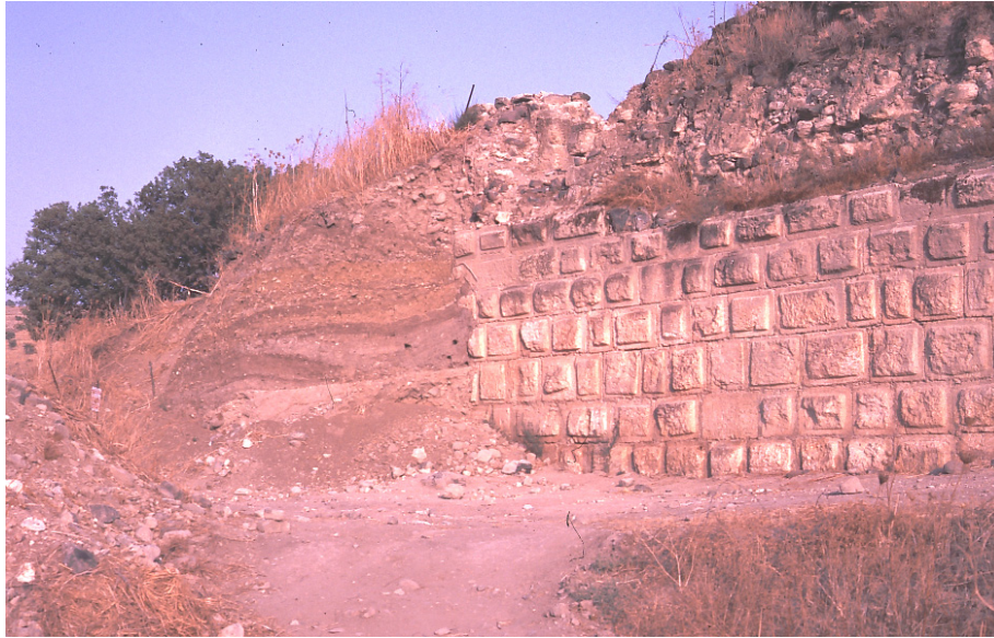
Figure 2: Northern Crusader defense wall built of meticulously hewn ashlars from a quarry on the hill to the west. On the left side is the construction ramp, which was used for hauling the blocks up to the high levels of the wall. The wall was actually buried as its construction advanced.
