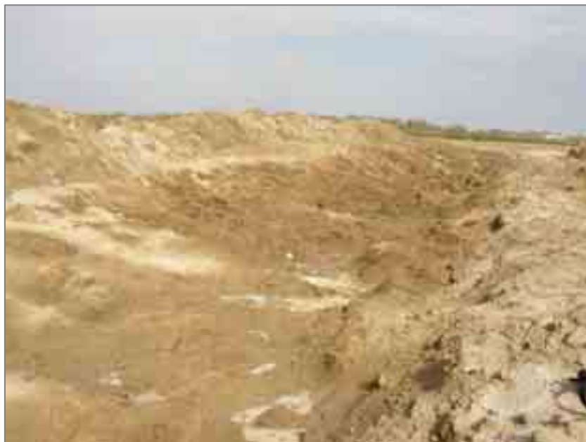
Photo 10. The artificial trench near the Qalya coast, where liquefaction and water injection occurred. Note the mud, water and cracks inside the trench. Photo was taken the day after the earthquake.
