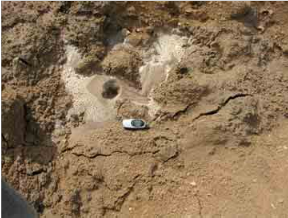
Photo 11. Mud cones and open cracks inside the artificial trench, near the Qalya coast. The cracks may reflect a very small scale lateral spreading. Photo was taken the day after the earthquake.
