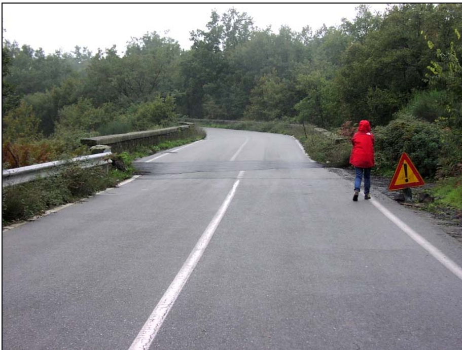
Figure f – Left-lateral faulting in the eastern slope of Etna volcano (Pernicana fault). Different segments of this fault move either by creep or stick-slip. More than half a metre of slip took place here during the october-november 2002 volcanic and seismic crisis. Photo E. Vittori
