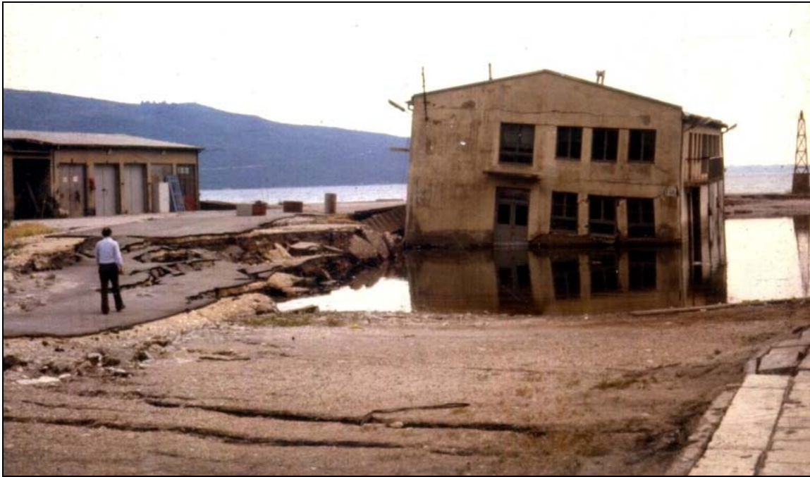
Figure q – Ground failure along the seacoast during the April 15, 1979 Montenegro earthquake ( M_w 6.9). Photo E. Iaccarino.
