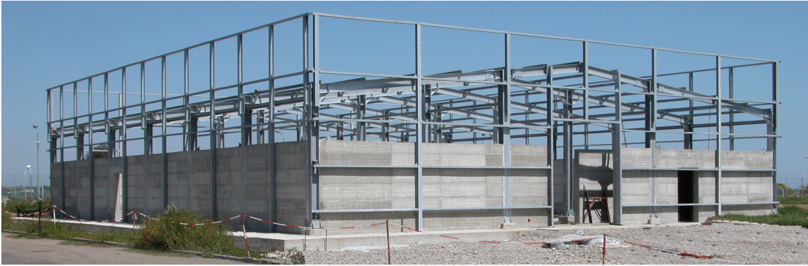
Figure 6: ITREC – The new storage facility under construction
