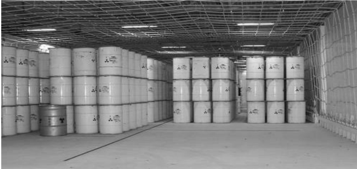
Figure 3: Caorso – ERSBA 2 storage facility
