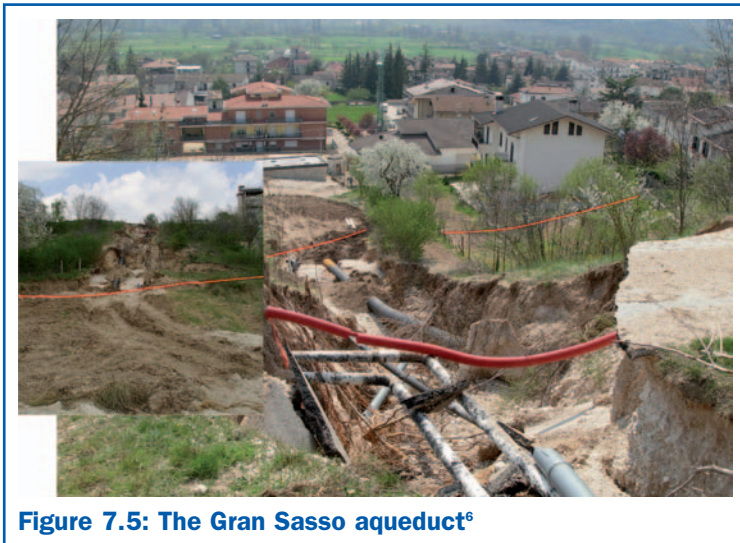
The Gran Sasso aqueduct restored, after the damages caused by surface faulting-induced displacement. The red line indicates the fracture caused by the earthquake of April 6 th 2009.
