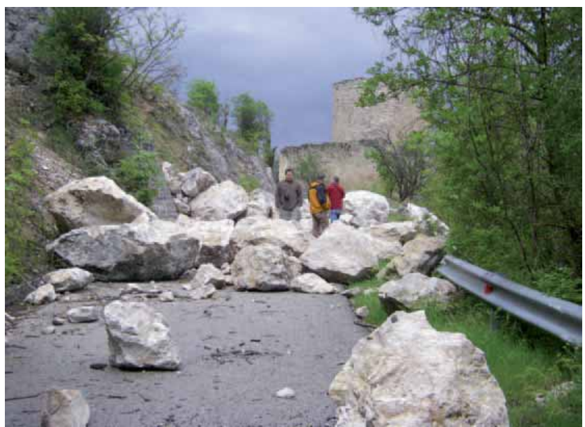
Figure 7.6: Landslide (fall type) near Fossa 7
