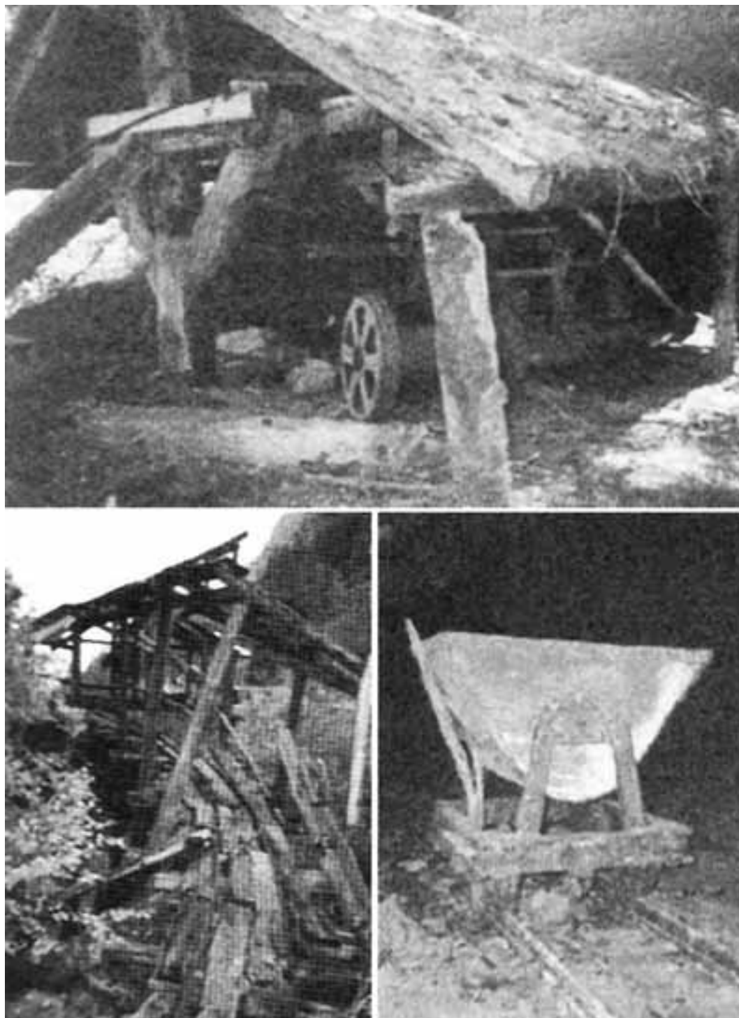
Figure 42 - Abandoned village and mine of Chuc. Workshop (top); terminal of the cableway (left); wagon at level 1331 m (right). Antique photographs in Lorenzini (1995).
