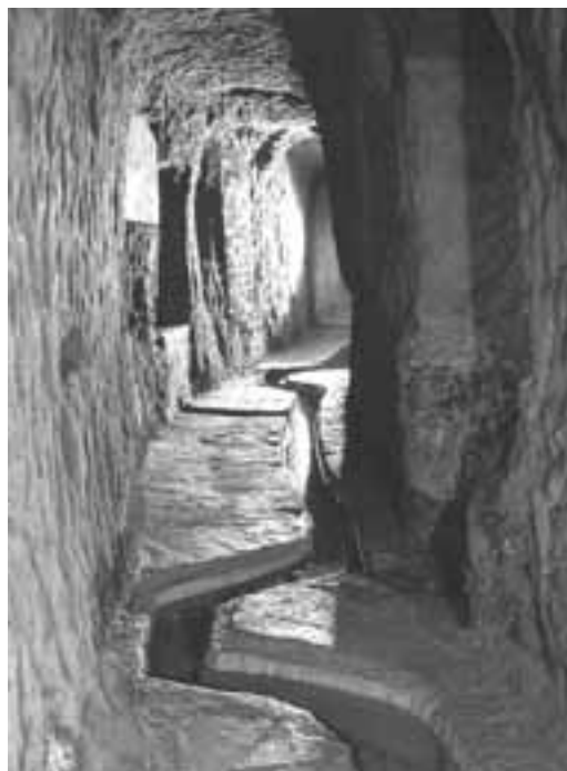
Figure 6 - Meandering path of a gorello to locally slow down and deepen water flow to ensure constant water distribution to intersecting gorelli of utenze (clients).
