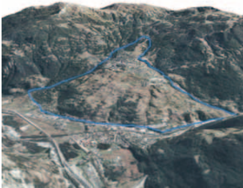
Figure 34 - Original frame of 1964 with the "Paleo-landslide".
