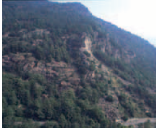
Figure 16 - Landscape view of the Pomeifrè rock fall area.
