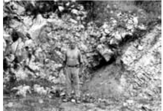
Figure 36 - Southeastern slope of M. Sparagio (Visicari). Intensely fractured Panormide Cretaceous limestones (left) above Serravallian shaly cover of the Trapanese Units.
