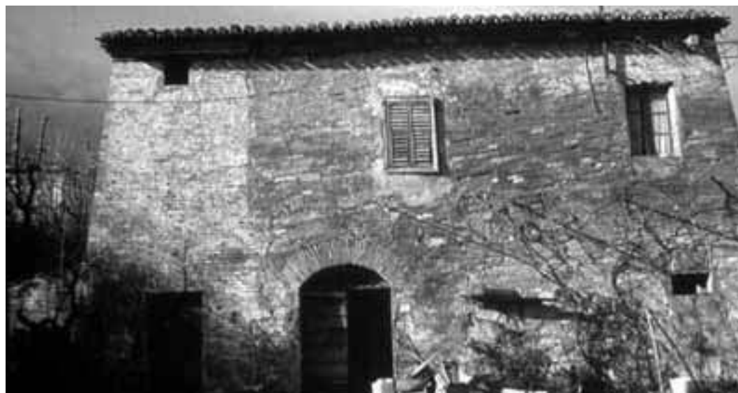
Figure 20 - A 16th century post-house, showing the cumulative effects of recurrent landslide movements on the Montagnolo slope.
