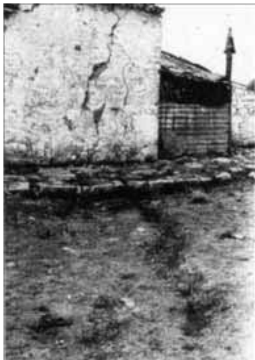
Figure 48 - Earthquake-induced ground fracture cutting a house
