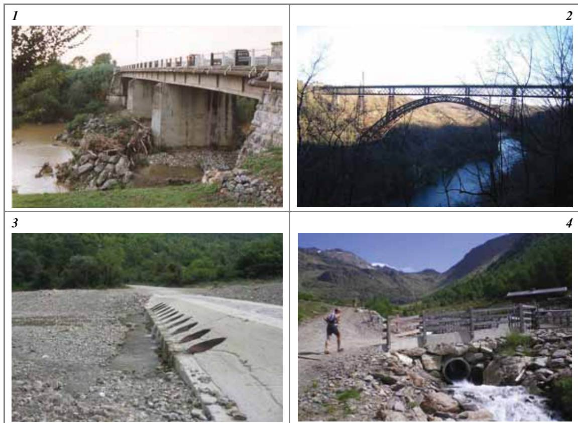
Figure 63 – Crossing structures. (1) Bridge with interference on fluvial dynamics; (2) crossing structure unrelated to the fluvial corridor; (3) ford with culverts; (4) culvert.
