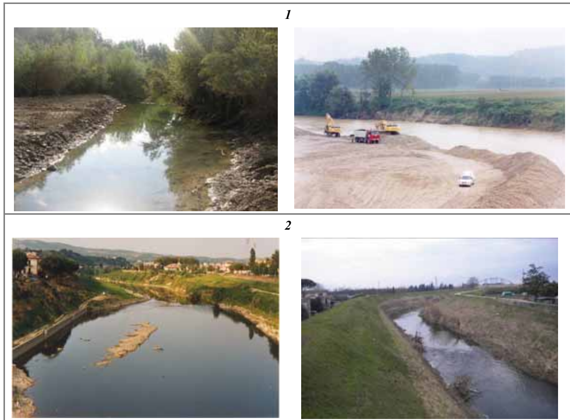
Figure 40 – Alteration of cross-section variability in semi- and unconfined channels. (1) Cases of partial homogenization of the cross-section due to interventions. (2) Cross-section homogeneity extended for long reaches due to excessive artificiality.
