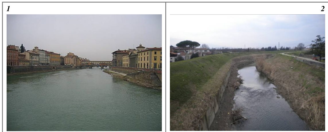
Figure 70 – Cases of bank protections plus levees in contact occurring for most of the reach (> 80%), for which a score of 12 is added.
