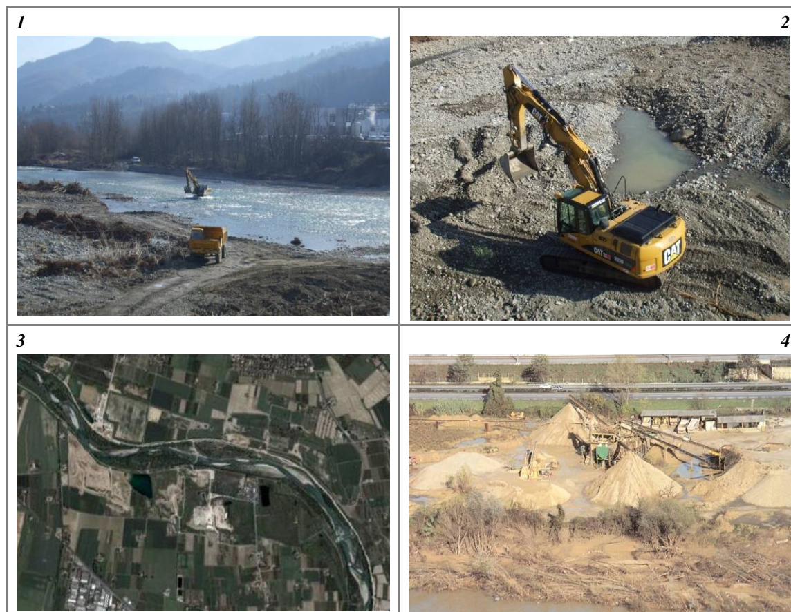
Figure 75 – Sediment removal. (1) and (2) Recent and present activity; (3) and (4) indirect indicators of intense past activity are the presence of mining sites. Assignment to Class B or C depends on the extension of the activity (localized or widespread), in the case of confined channels, and on the intensity of the mining activity either in the past and in recent times, in the case of semi- and unconfined channels.
