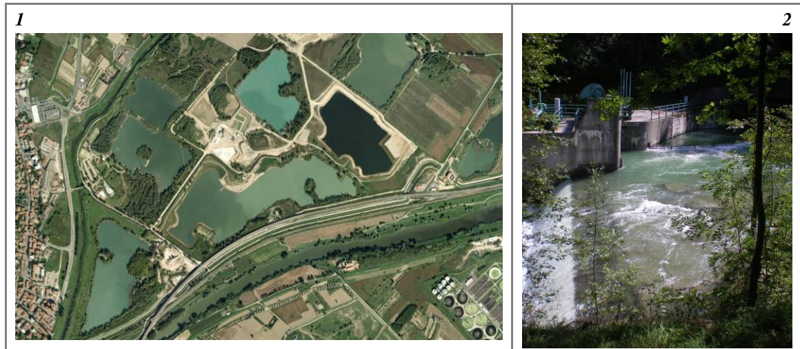
Figure 58 – Other structures (besides those defined for A1) that can cause an alteration of discharges within a reach. (1) Retention basins; (2) discharge abstraction.
