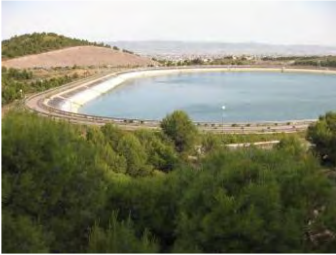
Figure 4.7: Irrigation pool situated nearby the epicentres of the 11 May earthquakes. Neither damage was observed in this area, nor instabilities on the talus on the background.
