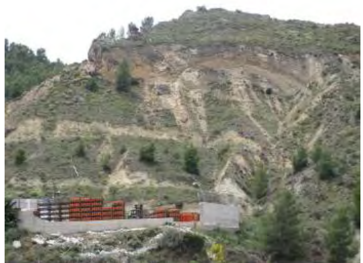
Figure 4.6: View of the slope enclosing a butane-gas storage site on the Pantano de Puentes road. No slope instabilities that could be attributed to the earthquakes were identified here, although the collapse of the concrete-brick wall is attributed to them.
