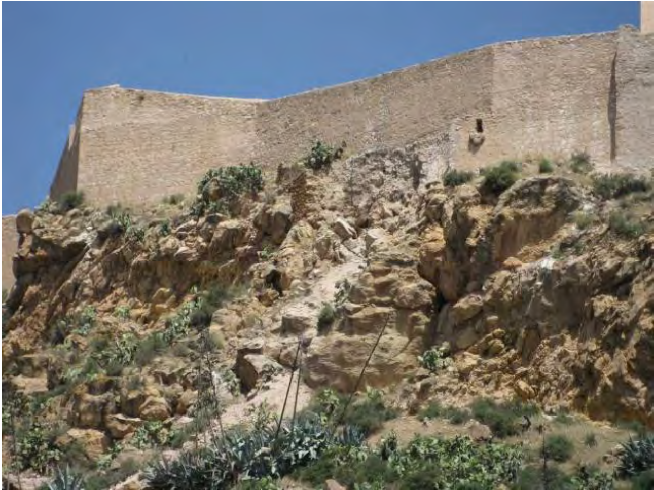
Figura 4.3.1: Collapse of an old retaining wall attached to the external wall of the Lorca's castle on its south face. This instability warned the dwellers of the houses situated right under the cliff, which asked us whether it was safe to return back to their places.
