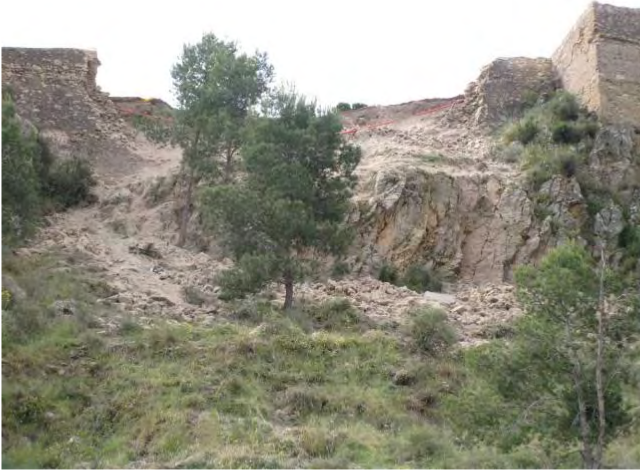
Figure 4.2.5: Collapse of the external wall of Lorca's castle (north face).
