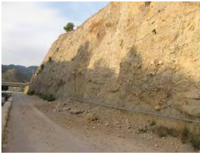
Figure 4.9: Shallow debris falls attributed to the May earthquakes on a service road of the Tajo-Segura canal.
