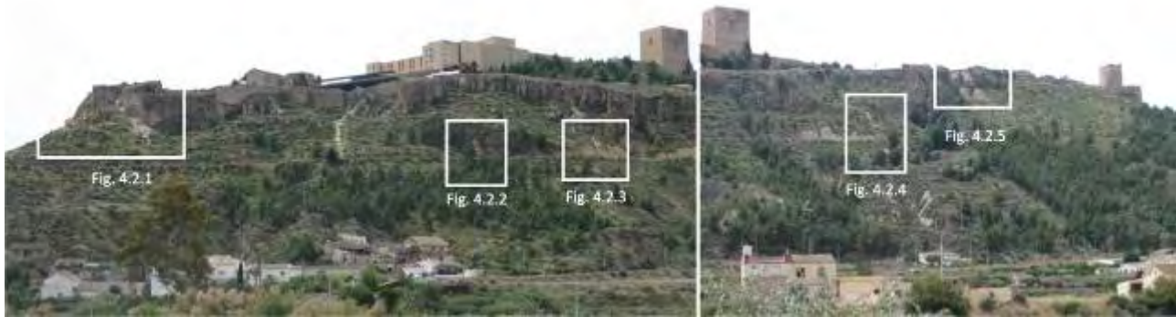
Figure 4.2.0: General view of the north slope of the Lorca's castle cliff. The most remarkable instabilities induced by the 11th May earthquake are identified.
