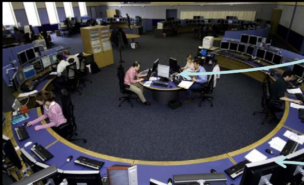
CITY CONTROL ROOM
