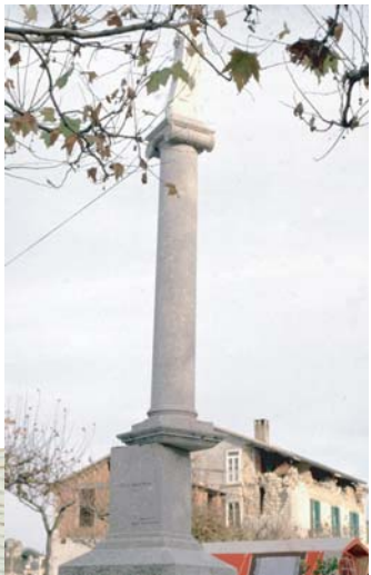
Fig. 17 - A historical parallel of the “Rocca del Gias” phenomenon: the rotation of a monumental column that took place in Pescopagano (Irpinia, Southern Italy) during the 1980’s earthquake (Photo F. Carraro).
