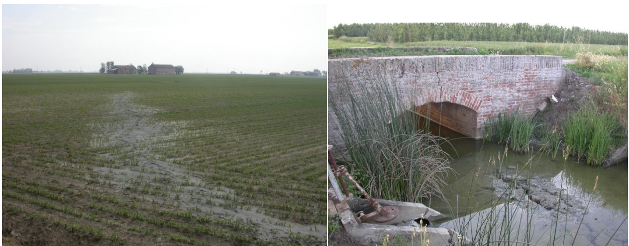
Fig.8 – Left: Scortichino, loc. Obici. Ground rupture with liquefaction . Right: Burana. Ground rupture with liquefaction in a channel
