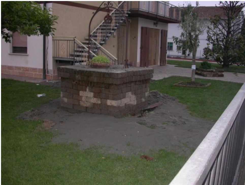
Fig. 9 – San Carlo (Sant'Agostino): sand ejected out of wells, most likely due to liquefaction
