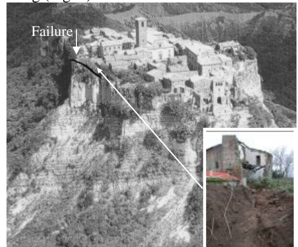
Figure 4. View of the northern side of the cliff and displaying of the large discontinuities.
