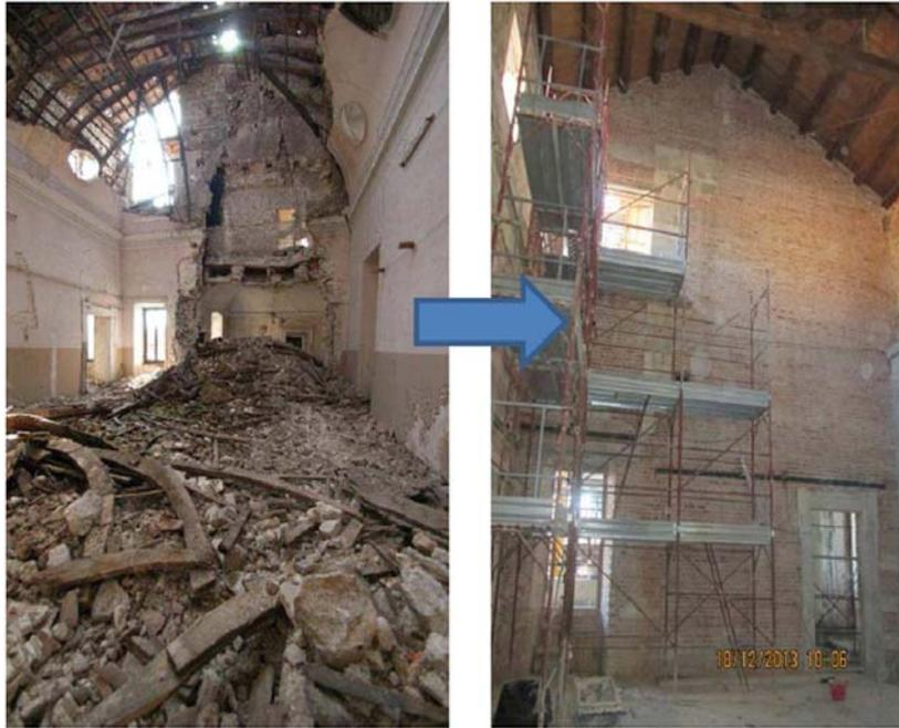
Fig. 75 - Reconstruction of the wall completely collapsed in a room on the main floor.
