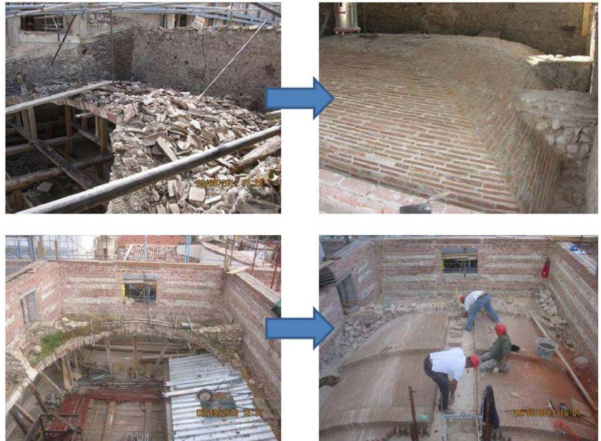
Fig. 76 - Main workings during the repair and consolidation of the damaged and collapsed masonry vaults.
