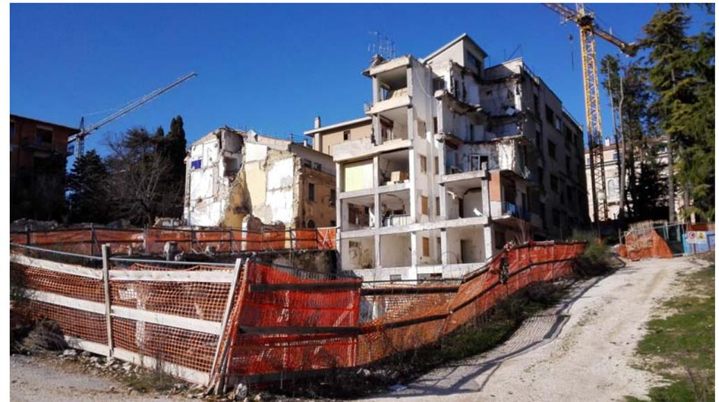
Fig. 64 - Example of RC building collapsed in Via Campo di Fossa during the April 6, 2009 main shock.
