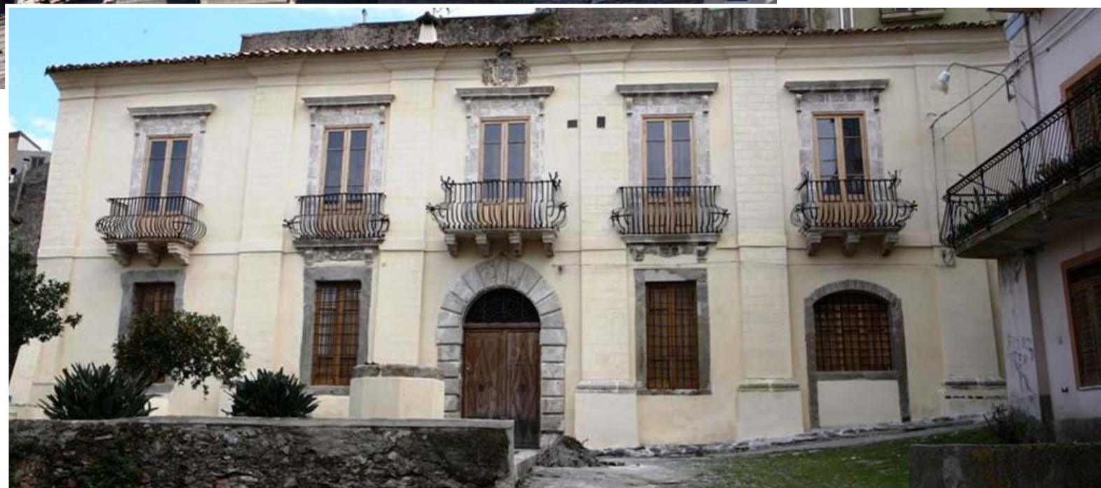
Fig. 1.20 - The Santa Lucia del Mela Medieval Hamlet. The façade of the Basile-Vasari Palace (XVII c.) with arches, doorposts and architrave of portals and windows decorated with Capo d'Orlando sandstones. Loc.: Santa Lucia del Mela. Central-Northern Peloritani Mts.
