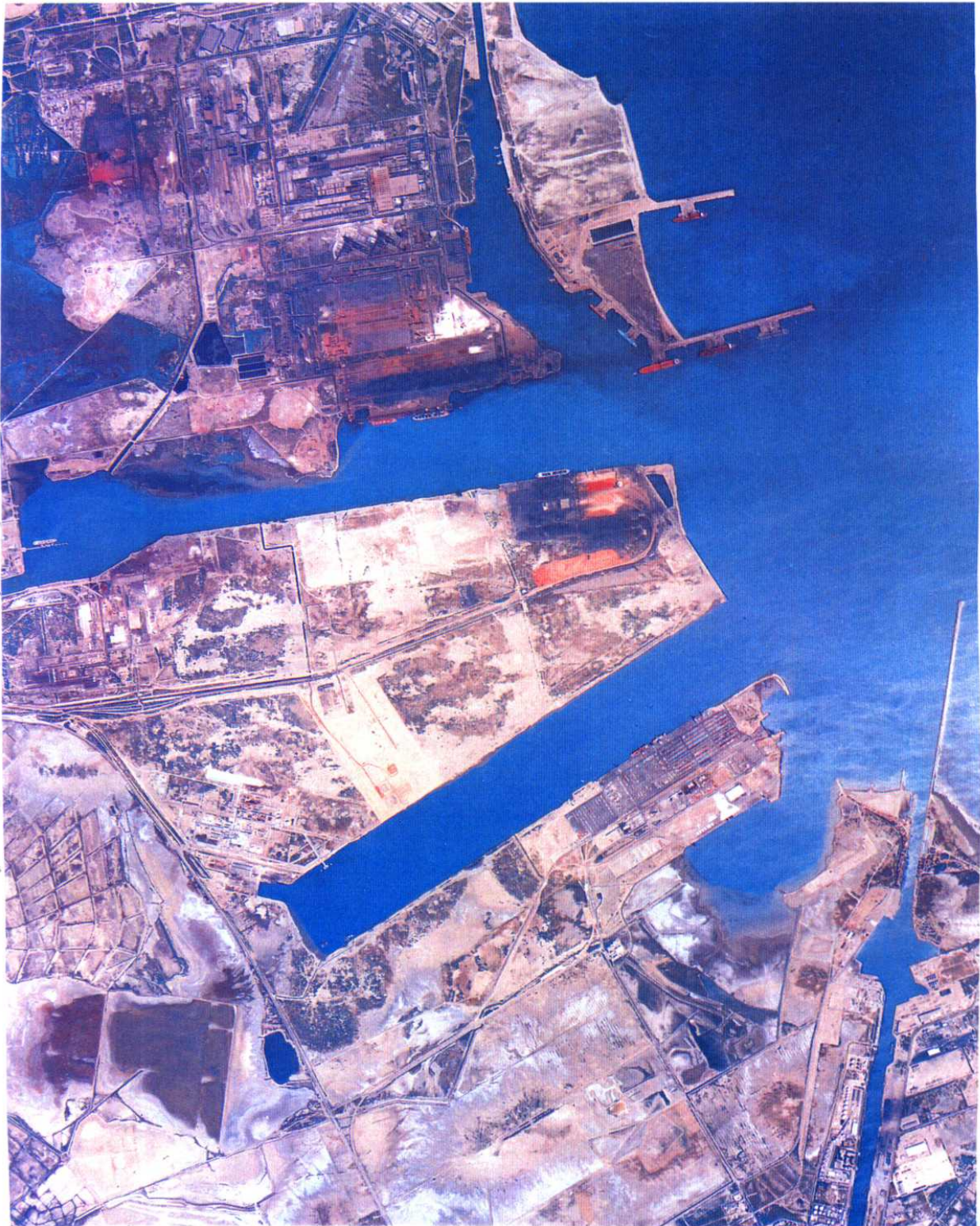
Photo 1 : A general view of the PMA access channel dredged (source : PMA).
