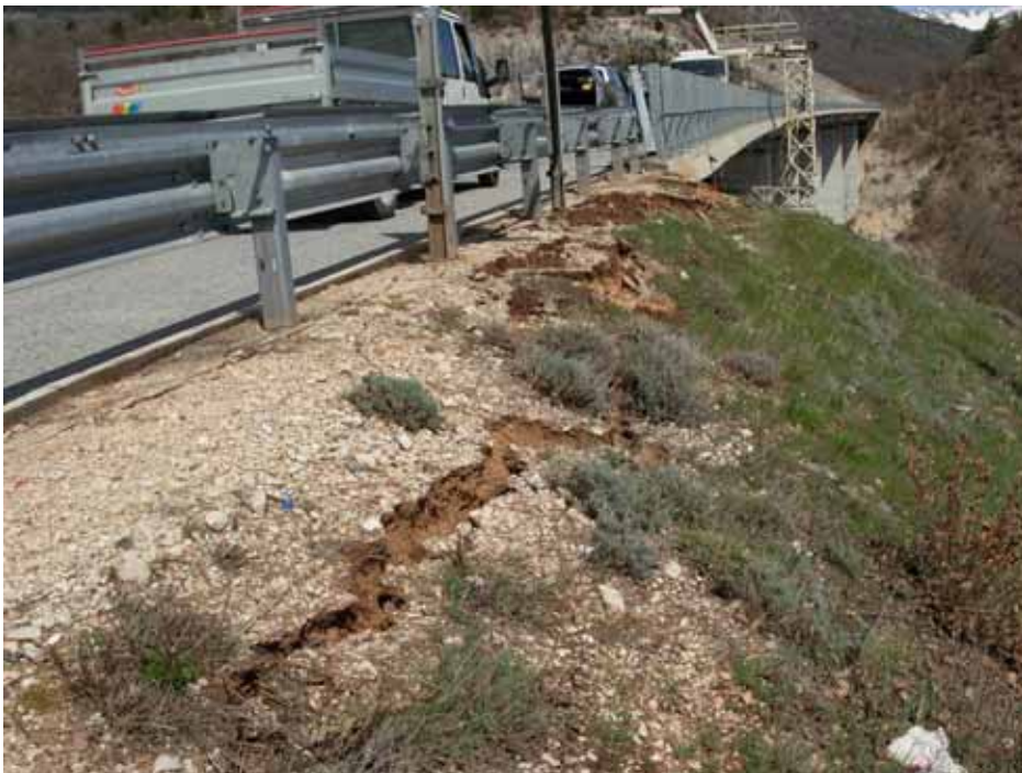
Fig. 34 – Above: Gravitational movement affecting the SS80 Road, km. 27,4. Below: A small landslide in artificial material along the Highway A24, between L'Aquila Est and Assergi
