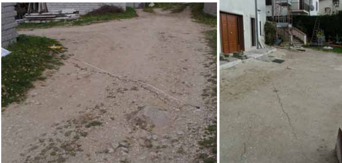
Fig. 9 - Ground ruptures between Tempera and Paganica
