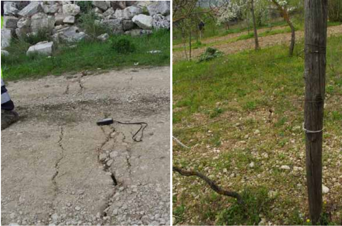
Fig. 10 - Ground ruptures in Paganica some tens of meters west of the broken aqueduct
