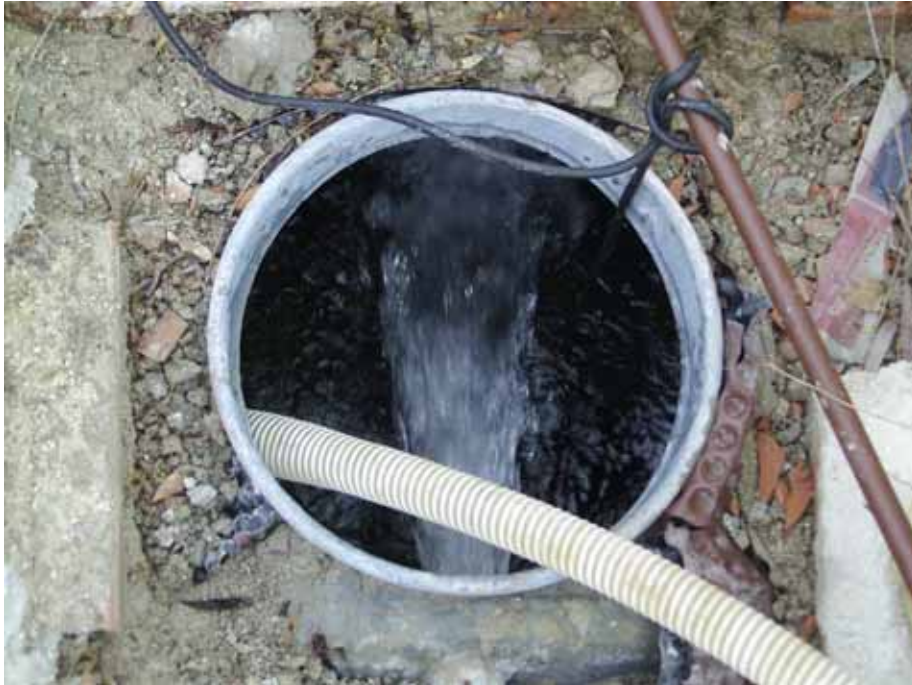
Fig. 42 – An increase in water discharge was recorded in local springs at Tempera
