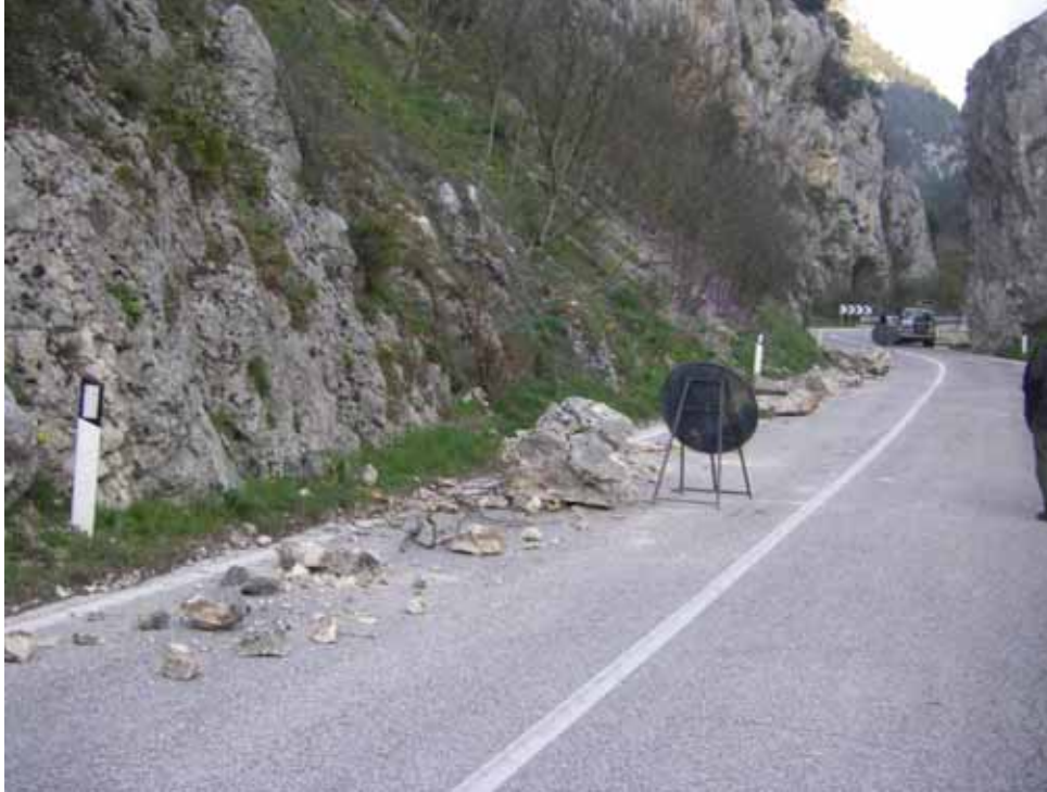
Fig. 30 – Rockfalls in the San Venanzo Gorges caused the interruption of the viability on the SS 17 Road.
