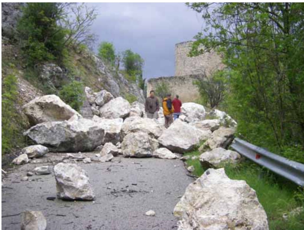
Fig. 29 – Fossa rockfall: huge boulders on a paved road.
