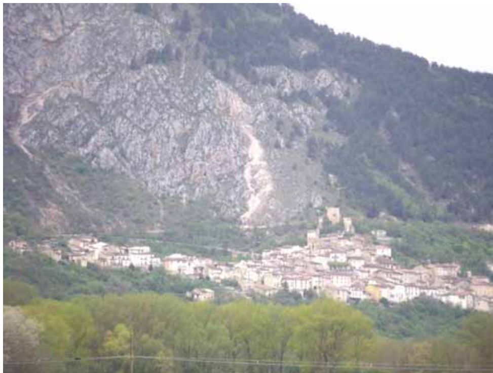
Fig. 28 – Panoramic view of the rockfall above Fossa
