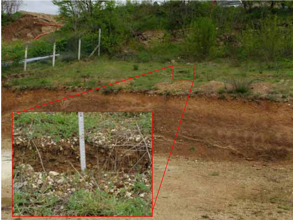
Fig. 12 - Ground ruptures in Paganica about 20 meters east of the broken aqueduct
