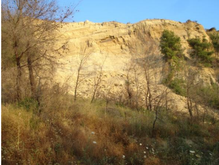
Figure 14. Slope movements like this one were observed in many sites at the epicentral area.
