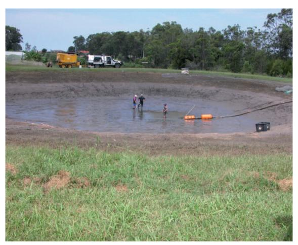
Figure 1. A small irrigation dam is pumped out before de-silting and REST removal - photo by Scott O'Keeffe, Queensland Department of Employment, Economic Development and Innovation
