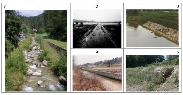
Figure 65 – Bank protections. (1) Bank walls (2) groyne; (3) rip raps; (4) gabions; (5) bioengineering bank stabilization.
