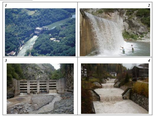
*Figure 55* – Transversal structures of alteration of sediment discharges in mountain areas. (1) Dam; (2) retention check dam; (3) open check dam; (4) sequence of stepped consolidation check dams.
