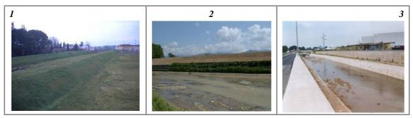
Figure 68 – Artificial levees. (1) Earth levees; (2) levee in contact with the channel; (3) bank walls with function of levees.
