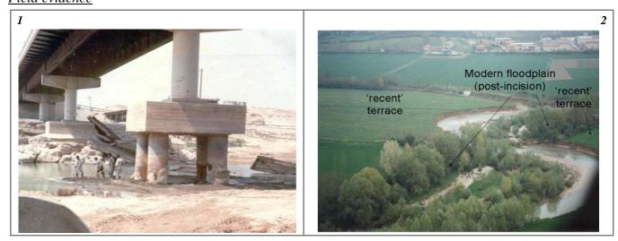
*Figure 81* – Field evidence of incision. (1) Exposed bridge piers. (2) Differences in level between modern (post – incision) floodplain and "recent" terrace (the latter corresponding to the pre – incision floodplain).
