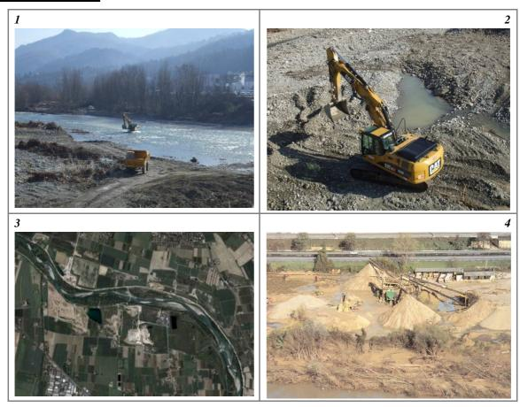
Figure 75 – Sediment removal. (1) and (2) Recent and present activity; (3) and (4) indirect indicators of intense past activity are the presence of mining sites. Assignation to  $Class\ B$  or C depends on the extension of the activity (localized or widespread), in the case of confined channels, and on the intensity of the mining activity either in the past and in recent times, in the case of semi- and unconfined channels.
