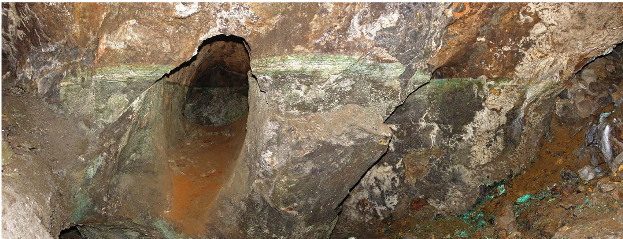
Fig. 36 – Upper part of an old excavation opening showing encrustation of chrysocolla and gypsum.
