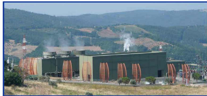
Geo-thermoelectric power plant
