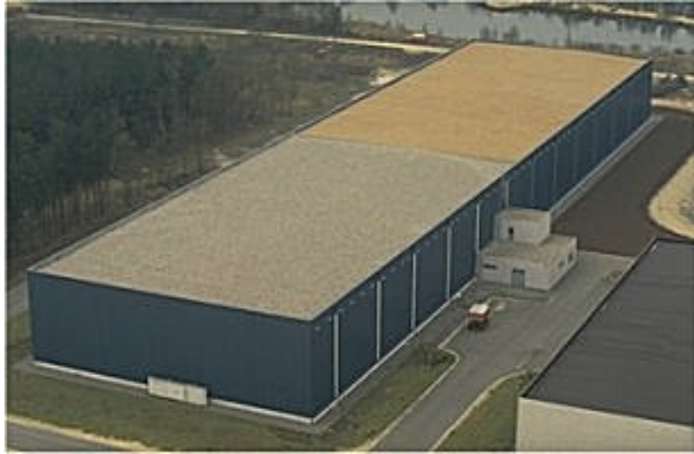
Figure 8: Project of the Latina NPP recently licensed new interim storage facility
