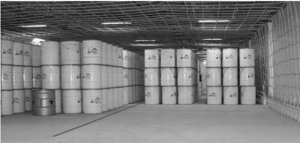
Figure 3: Caorso – ERSBA 2 storage facility
