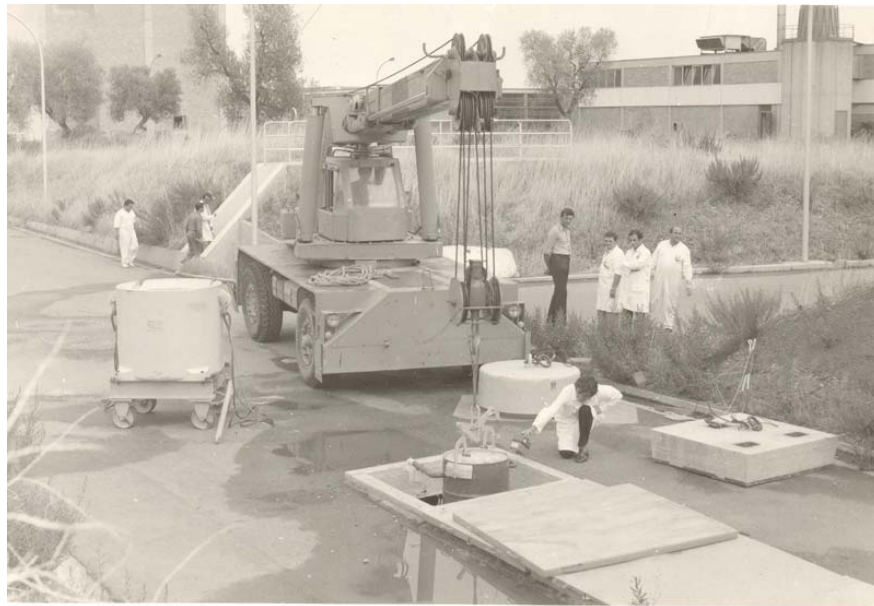
Figure 9: Historical picture of burial of radioactive waste in pits at the ITREC facility in the years '70s.
