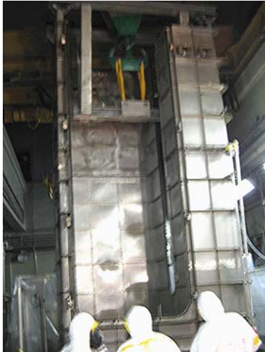
Fig. 1. Metal basin 5 m long during extraction from EUREX SFP.
