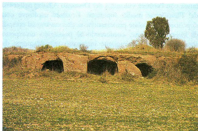
Fig. 2. – Galleries mined in the “pozzolanelle” ignimbrite. Similar structures are frequent in the Tor Marancia area, particularly in those sectors intensively exploited by mining in the Roman and in the Middle Ages.
