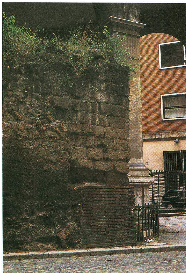
Fig. 3. – A) Serviane Walls, built with blocks from the “pisolithic tuff”, present in Via Salandra, close to Termini railway station. B) Natural outcrops of the “pisolithic tuff” in the Tor de’ Cenci area, south of Roma.
