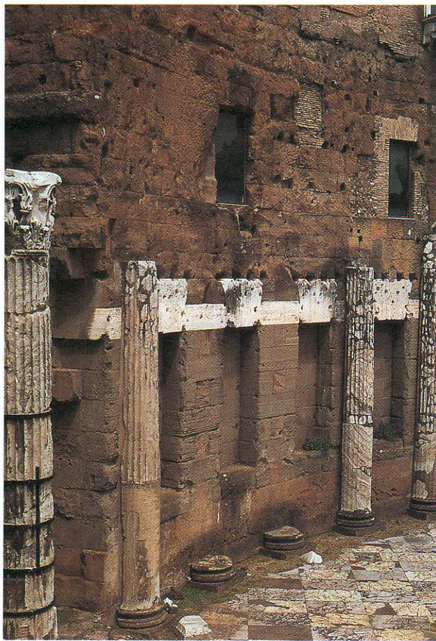
Fig. 7. – Foro di Augusto. This forum was largely created using "lapis Gabinus" and the "lionato tuff".
